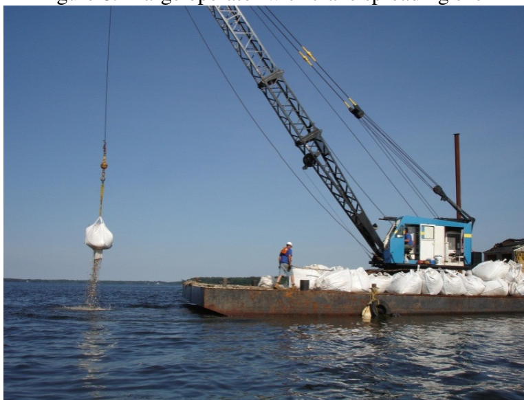
Figure 8. Barge operator with crane spreading shell
