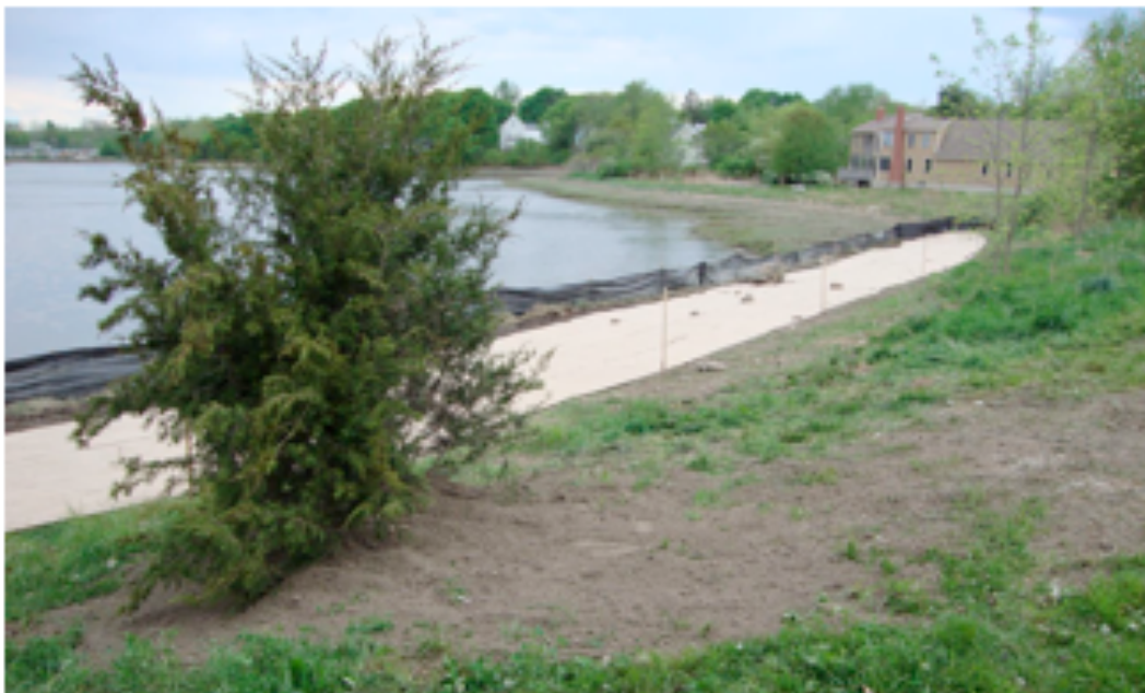
Figure 3. Burlap covering exposed soils in work area; red cedar replanted on upland. Picture taken on May 5 th , 2010.
