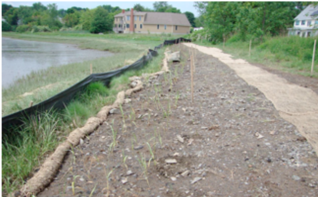
Figure 5. Planting and site work complete, June 5 th , 2010.
