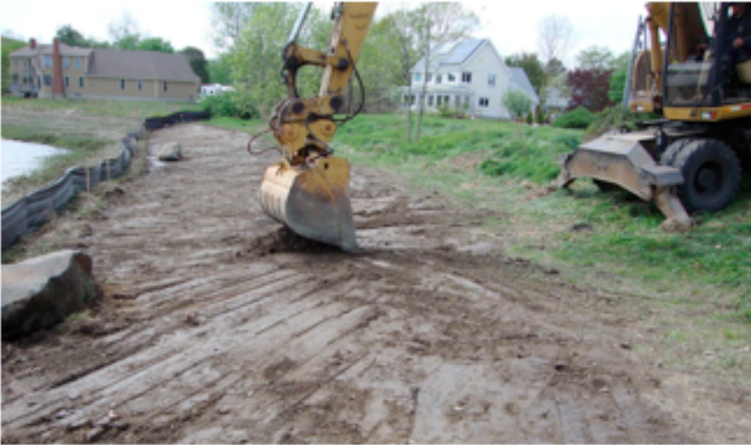
Figure 2. Re-grading the shoreline. Note that two large rocks were replaced at the site.
