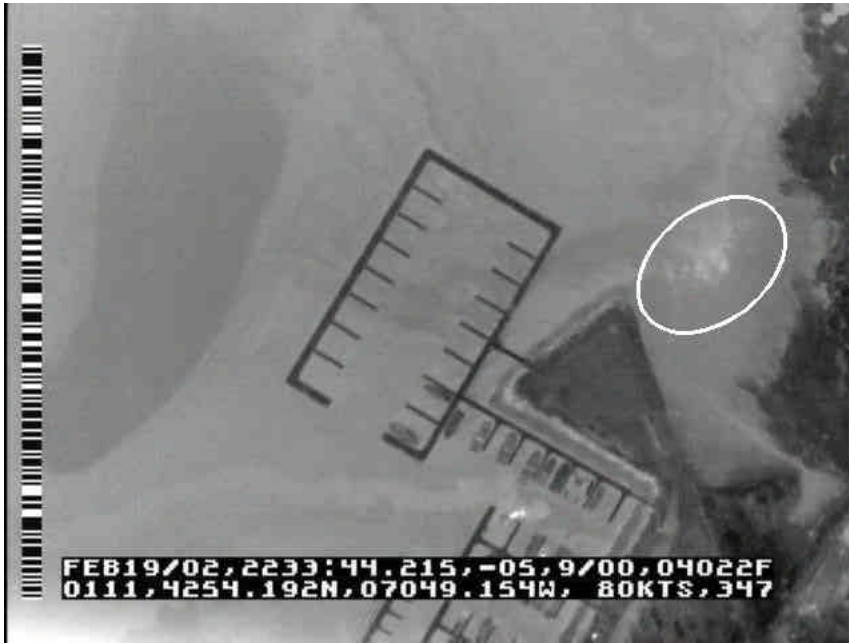
Figure 12:Groundwater Discharge Location HH0057.1.3
