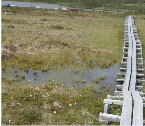
Fig. 1: Boardwalk on Stordalen Mire that is sinking due to thawing permafrost
