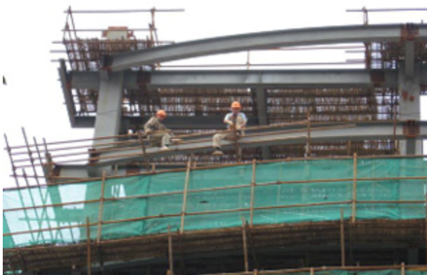
New supported by the old: in Shanghai, bamboo scaffolding is used for construction of modern high-rises (Susannah Pratt.)
