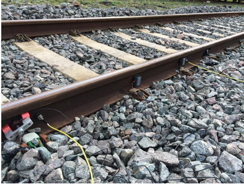
Figure 6-10: Installation of accelerometers and AE sensors on the track
