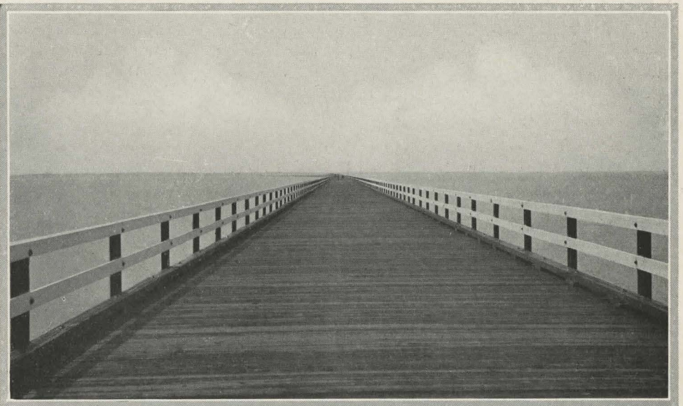
ST. AUGUSTINE-GREEN COVE SPRINGS BRIDGE, FROM MID-RIVER TOWARD CLAY COUNTY
