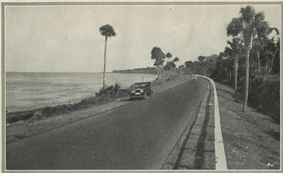
DIXIE HIGHWAY, SOUTH OF MELBOURNE, ALONG INDIAN RIVER
