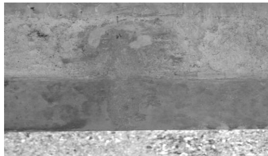
Figure 3-7: Finished repaired section
