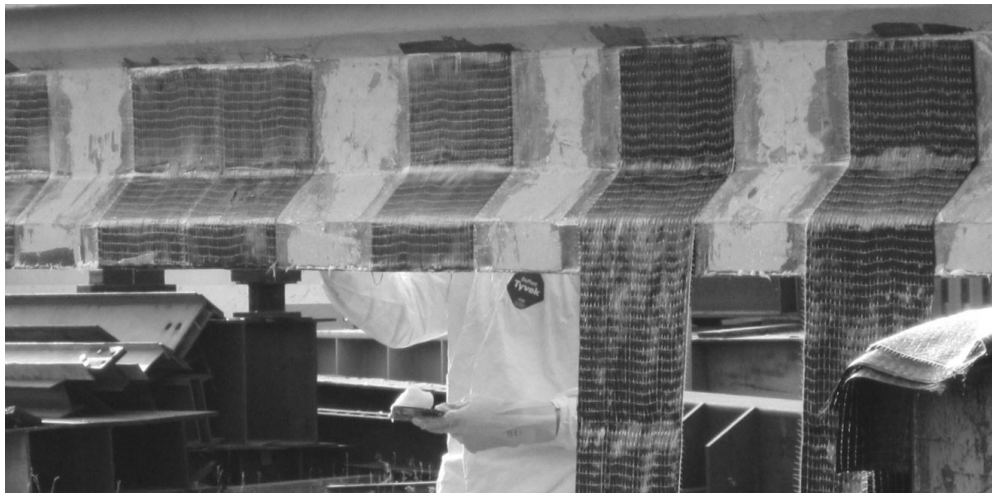
Figure 3-15: Transverse CFRP U-wrappings being applied by FIBRWRAP
