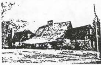
OLD FAIRBANKS HOUSE. BUILT 1636
