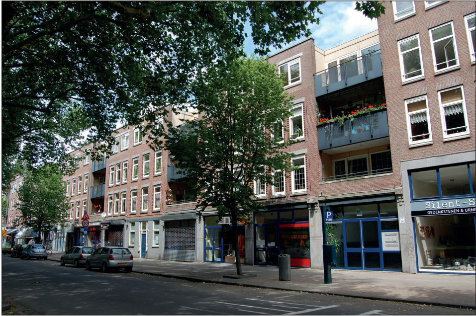
Fig. 5. Saved from demolition Source: own
