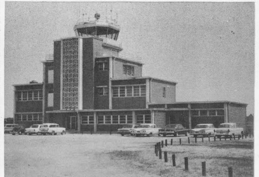
AIRPORT CONTROL TOWER
