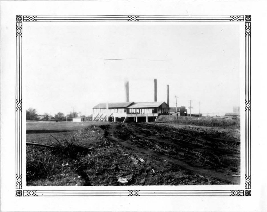
REFUSE INCINERATORS in action at the PALM STREET SITE
