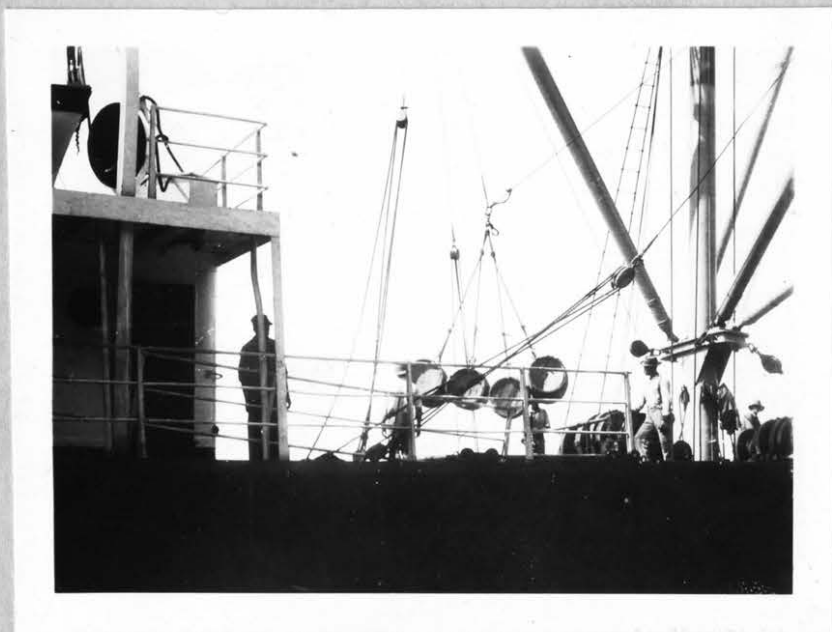
Most of loading and unloading at MUNICIPAL DOCKS is done with ship's tackle. Loading rosin for export.
