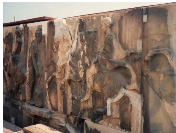
(16) Sculptures damaged by pollution still in situ on the Parthenon
