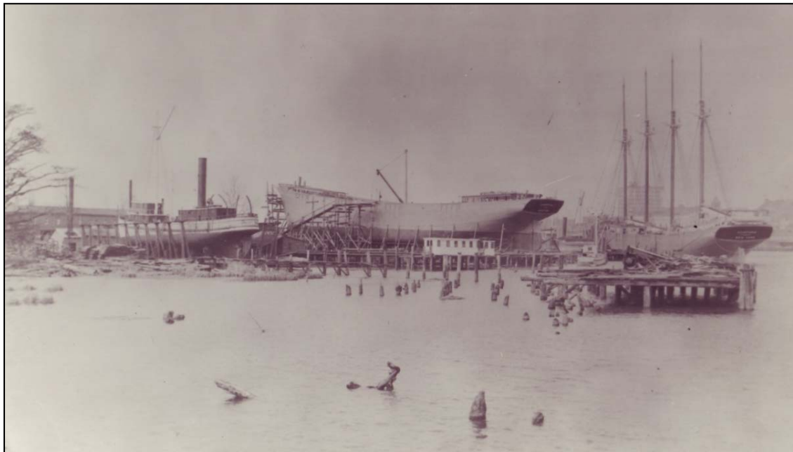
Figure 3-6 Hoppague and Commack under construction on Eagles Island (Image Courtesy of the North Carolina Underwater Archaeology Branch).
