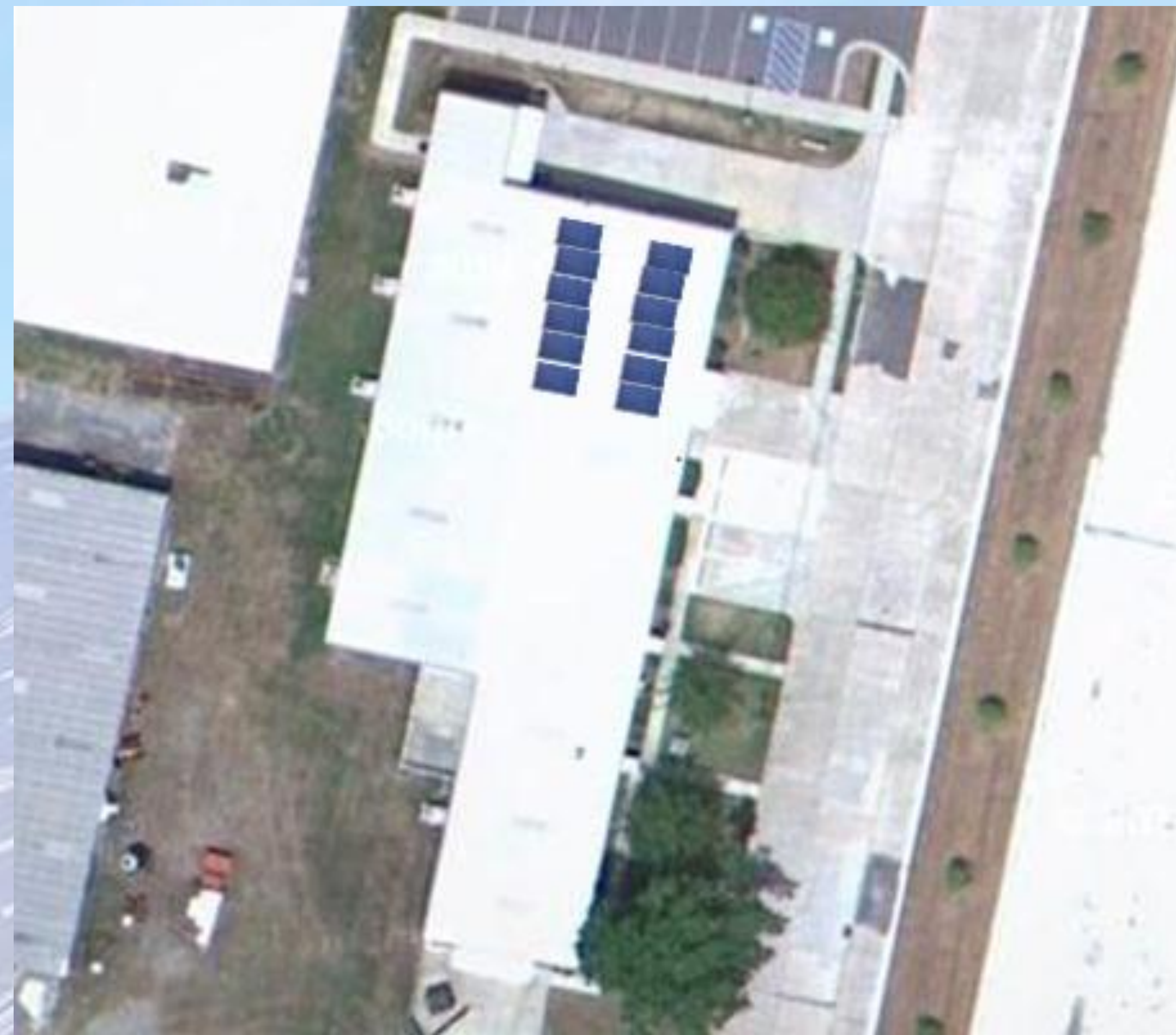
Figure 8: Proposed solar panel installation. This image shows potential roof area required and how the solar panels would be placed on the structure.
