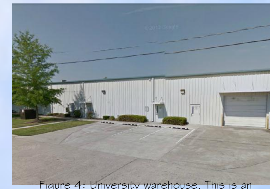
Figure 4: University warehouse. This is an exterior photo of the proposed warehouse for solar panel installation.
