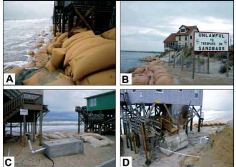
FIGURE 12. Photographs of sand-bagged houses in South Nags Head on Bodie Island (Panel A) and Bogue Inlet on Bogue Banks (Panel B) demonstrate the loss of the public beach. Photographs of sand-bagged houses in South Nags Head on Bodie Island (Panels C and D) with exposed and broken septic tanks and drain-fields. After storms these houses are condemned until the septic systems can be temporarily repaired and reburied in sand. Photographs are by S. Riggs.
