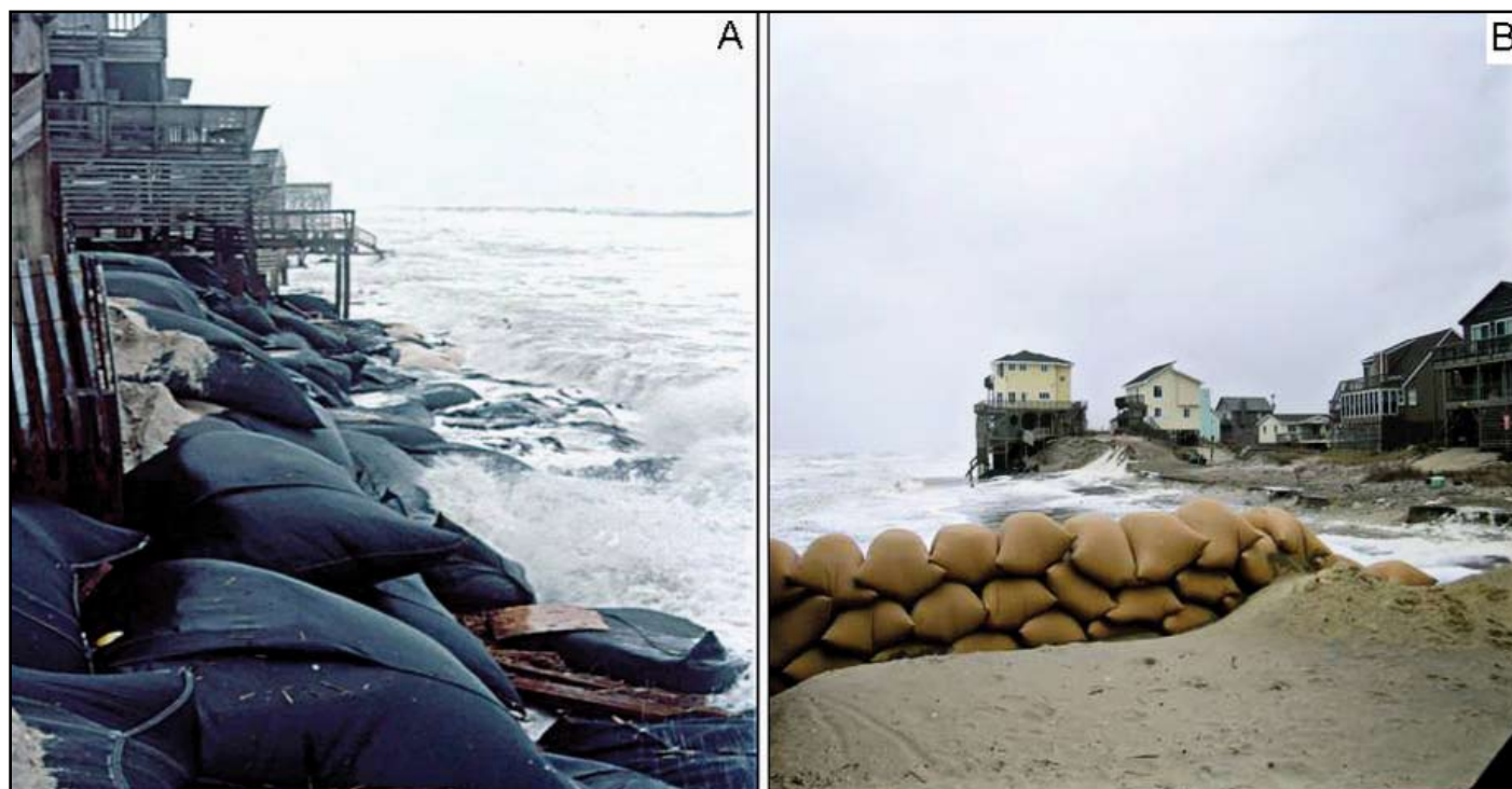
FIGURE 18. Panels A and B show the South Nags Head shoreline hardened with sand bags. Loss of the beach has left houses in the surf zone. Severe lateral erosion has also resulted, thus jeopardizing adjacent access roads and houses. Photographs are by S. Riggs.
