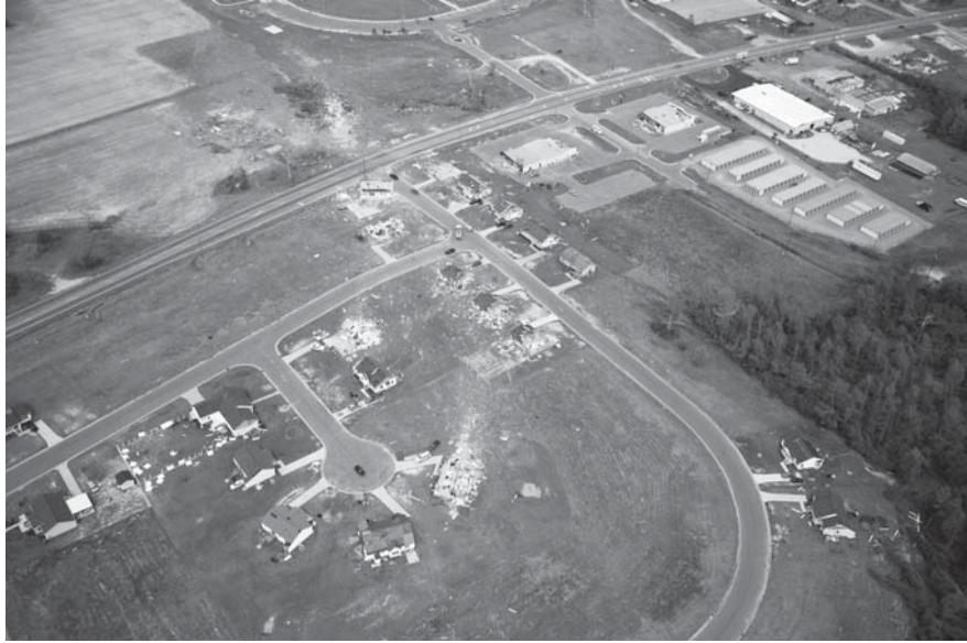
Figure 17. Aerial photo of EF3 damage to the neighborhood along Highway 13. View is to the northeast. Highway 13 runs left to right (courtesy of the National Weather Service).
