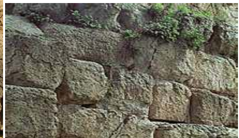
Detail of wall (Plate 18)
