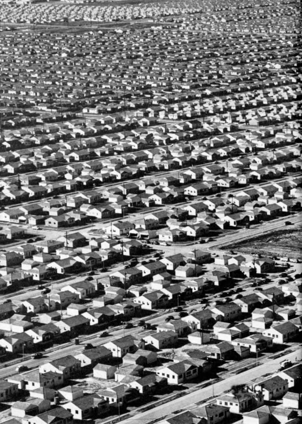
A small portion of Lakewood area of new homes. Total area covers five square miles, 26,000 homes.
