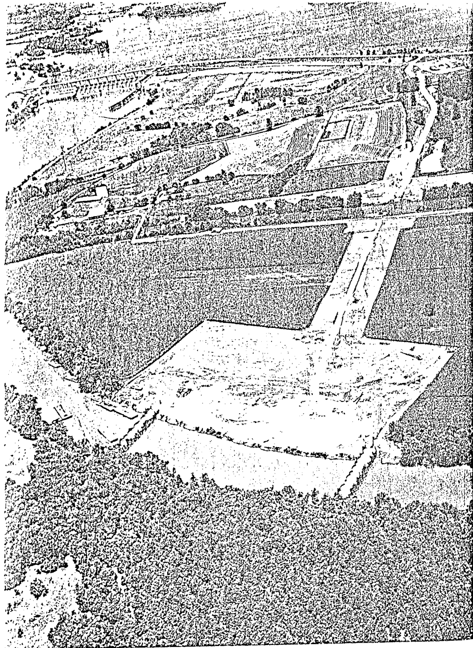
This view shows preliminary construction activities at the site of the Tellico project on the Little Tennessee River, which was started late in the fiscal year. The Tellico Dam, for which the site is being cleared, will extend navigation 33 miles upstream on the Little Tennessee River to areas favorable for industrial development. An 850-foot-long canal will connect Tellico reservoir with the reservoir of Fort Loudoun Dam, shown in the upper left background, and the two installations will be operated jointly to provide navigation, flood control, and power.
