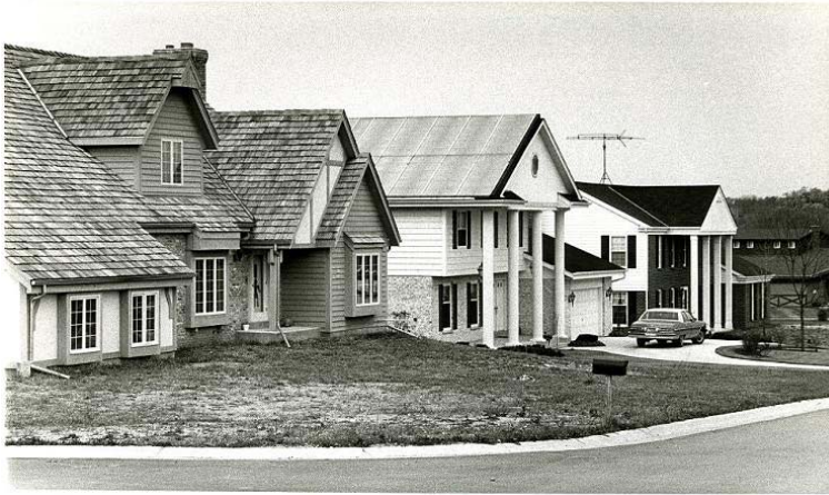
Pic 3: Photograph of the Prah house with solar panels and the adjacent Maretti house.
