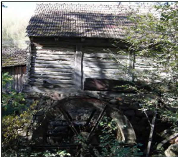
Fig. 8. Water mill from Vărciorog village
