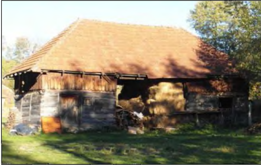
Fig.. 5. Barn, shed and chicken coop facade (Valea Crisului, Bratca commune)
