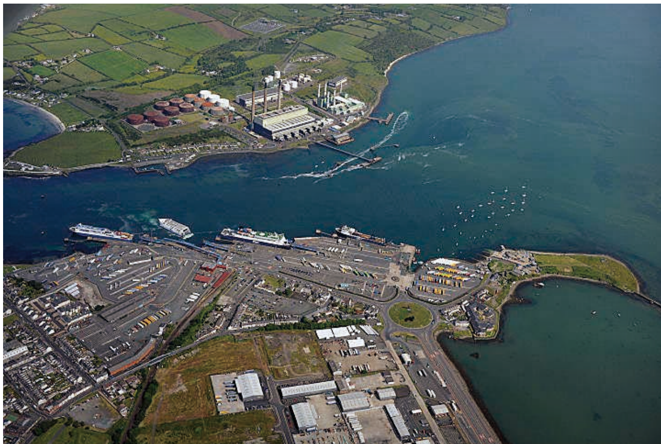
FIGURE 14. AERIAL VIEW OF PORT OF LARNE.
