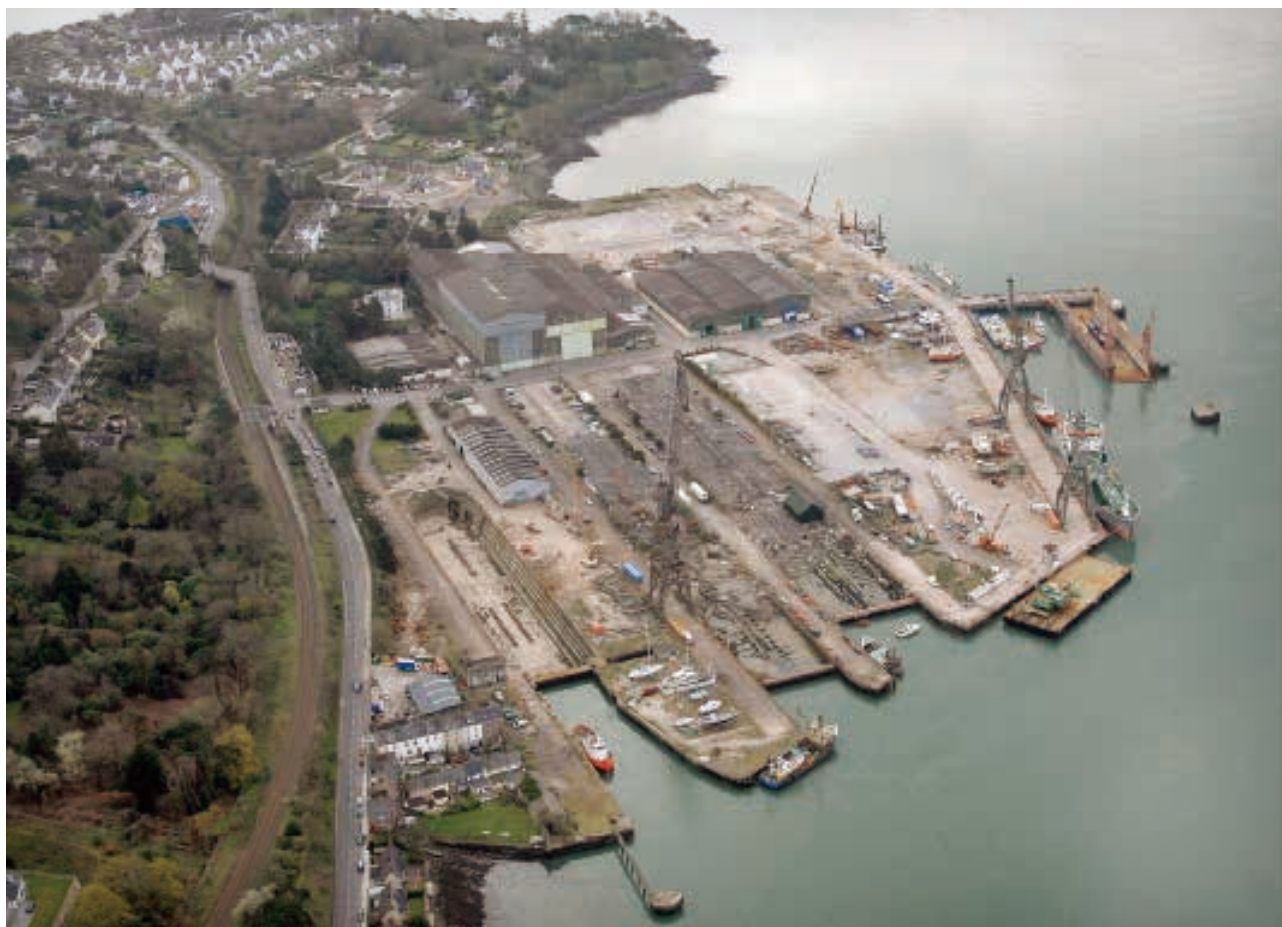
FIGURE 8. AERIAL VIEW OF CORK DOCKYARD.
