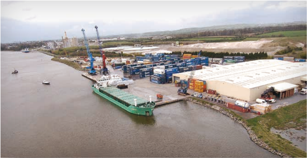
FIGURE 2. DROGHEDA PORT – TOM ROES TERMINAL.
