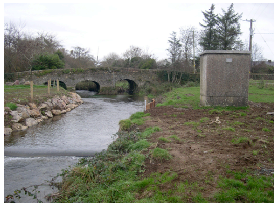
Figure 4. Station at Goff's Bridge.
