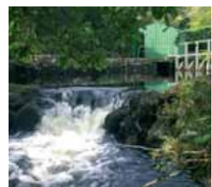
Below the Mill Race Trap Falls - Marine Institute, Newport Facility
