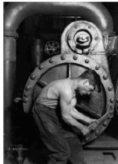
Image by: Lewis Hine, Power house mechanic working on steam pump , courtesy of the National Archives and Records Administration, 1920
