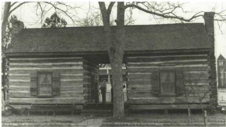
13. Cornelius Lynch House, Stewart County, Georgia, built 1848. Both the log construction and central breezeway "dogtrot" plan are thought to have originated with Delaware Valley Finno-Swedes. (Photo by author, Shaping Traditions )
