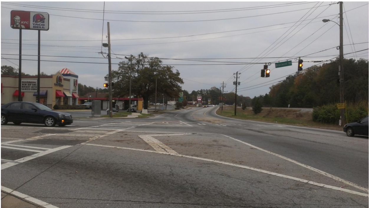
Figure 31 View of Hotspot 8
