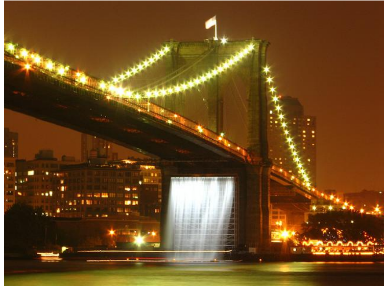
Figure 8. Example of a site-specific installation.
