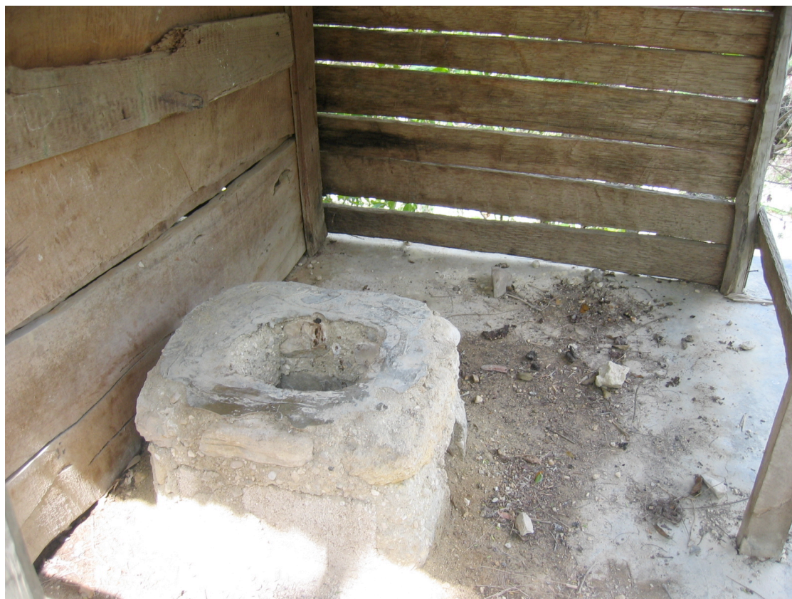
Figure # 14: Latrine at St. Pierre, Grand Bois, Haiti
