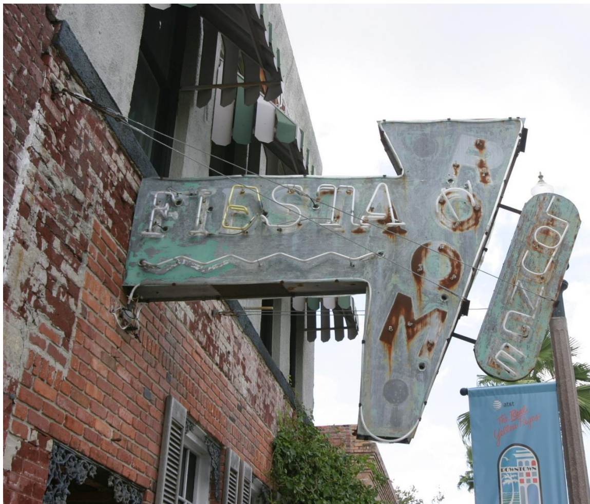
Figure 2: Original sign hanging in front of The Fiesta Room Lounge 75
