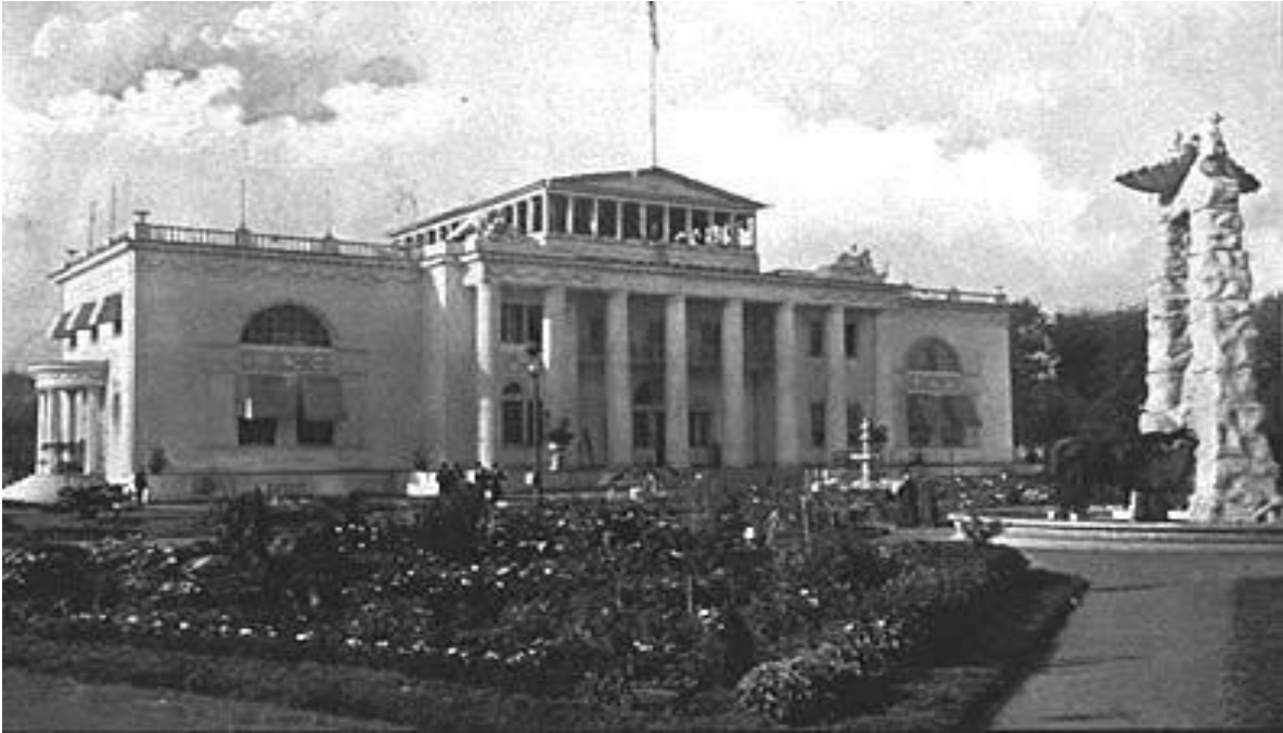
Figure 12. Women's Building at the Centennial Exposition of 1897. (Photo Courtesy Metro Nashville Tennessee Parks Board).
