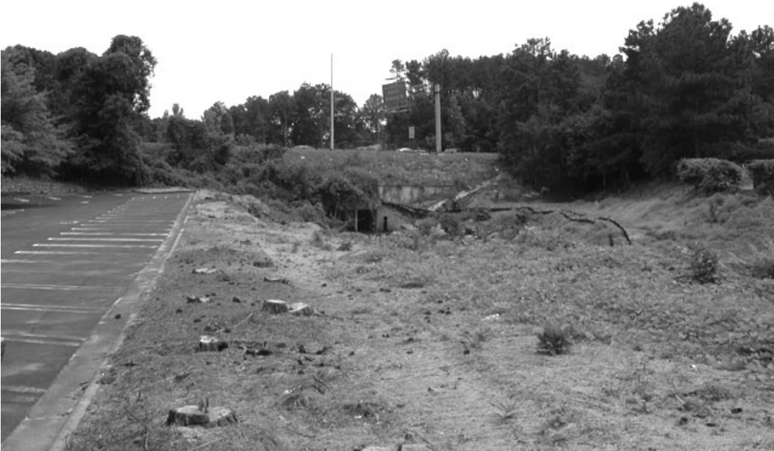
Figure 17. Southern site of “fly-over” bridge at I-285, 2005 Source: Author
