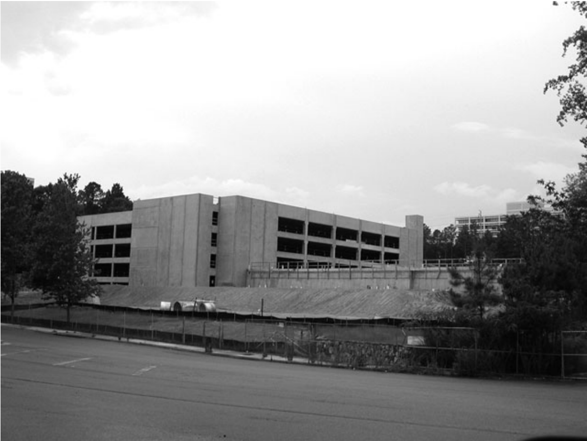
Figure 13. New construction at the same site as Figure 12, 2005 Source: Author
