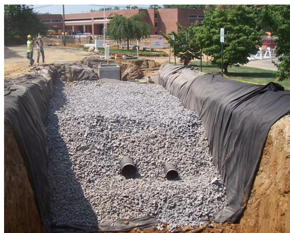
Imagen 4. Trinchera (Fuente: Center for Sustainable Communities: http://www.csc.temple.edu/tvssi/images/survey_BMP/delaware_countycc/dccc_2008_infiltration_tren.jpg )
