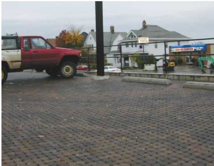
Imagen 38. Pavimento permeable en adoquin en St. Germain's – Diamond-Vogel Parking Lot, 17th Ave East & London Rd Duluth, Minnesota (Fuente: Lake superior Streams: http://www.lakesuperiorstreams.org/stormwater/toolkit/pervPaveCase.html )
