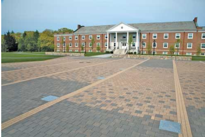
Imagen 37. Pavimento permeable en adoquin en Stonehill private Catholic liberal arts college, Boston (Fuente: Land Scape Online: http://www.landscapeonline.com/research/article/15100 ).
