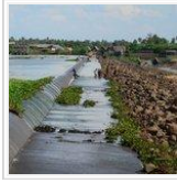
The water storage problem
