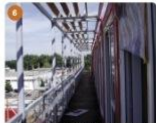
6 External walkways provide access to the individual homes;
