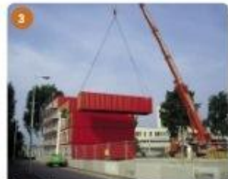
3 Standard transportation and easy to stack and connect;
