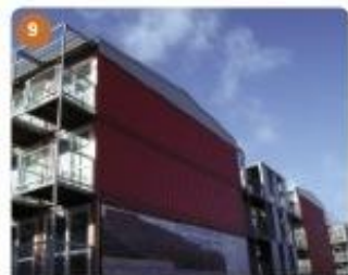
9 Additional roof for increased insulation and rainwater handling;
