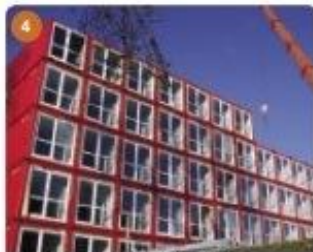
4 Building up to seven levels possible without additional structures;
