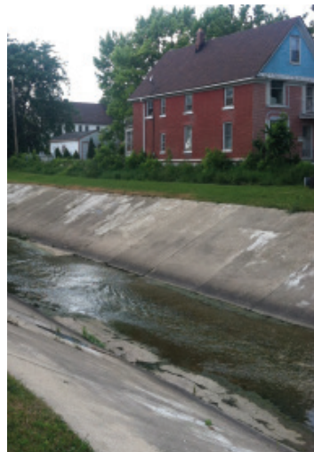
BEFORE: This picture of the Kinnickinnic River is representative of what the river looked like before the naturalization effort expanded the banks of the river, allowing it to meander. Photo courtesy of the Sixteenth Street Community Health Center.
