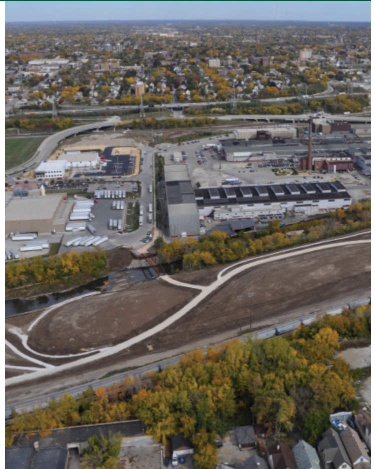
A bird's eye view from fall 2012 of the old Milwaukee Road rail yard during restoration, now reconstructed into the Three Bridges Park along the Hank Aaron Trail. Photo courtesy of the Redevelopment Authority for the City of Milwaukee.
