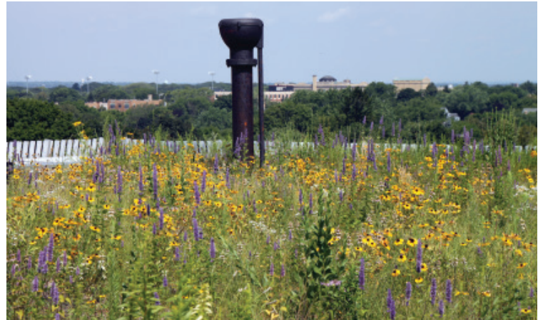
The native prairie green roof on top of the Sandburg Commons. Green rooftops can absorb rainwater, slowing the time it takes for the water to reach the sewer system and helping the sewer cope with heavy rain events. Photo courtesy of Jim Wasley.
