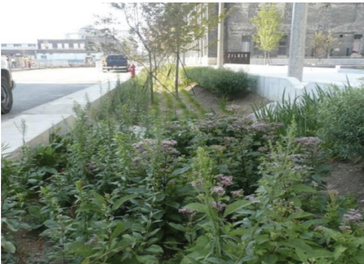
In the renovated neighborhood, bioswales filter water into a 250,000 gallon reservoir below ground, delaying flood water from entering the town's stormwater system. The native plants are also both drought and salt tolerant—important in a cold climate where salt builds up in the streets over the winter. Photo courtesy of Zilber Ltd.
