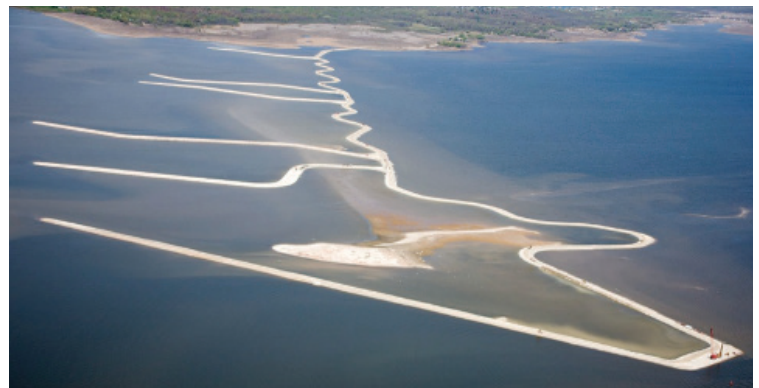
The wave barrier connected to the outline of Cat Island, June 2013. The fully constructed shell for the island chain will protect the wetland habitat on shore. Photo courtesy of the Army Corps of Engineers.
