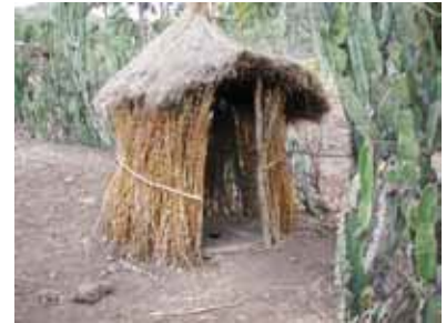
Innovative very low cost "Arborloo" toilet in Harbu. After a year or less of use the slab and superstructure are moved to a new location and a tree seedling is planted on the pit. Tsegahun Tessema for CRS.
