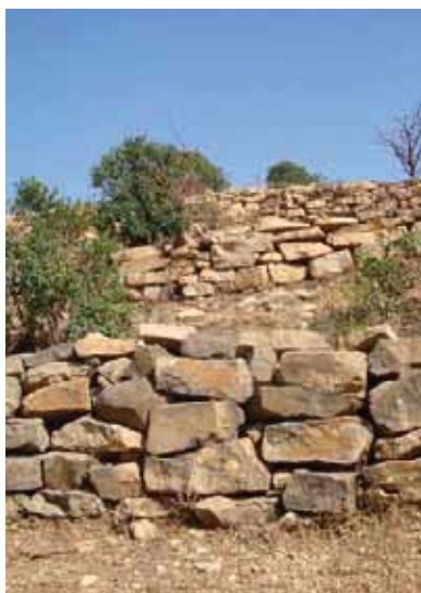
Rock terraces to control soil erosion, an example of natural resource management in Legedini. Paul Hebert for CRS.
