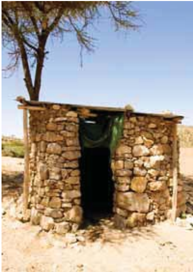
An Arborloo ecological toilet with a rock superstructure, Legedini. Rock is abundant in Legedini and this dry-stack rock superstructure is easily and quickly constructed. Paul Hebert for CRS.
