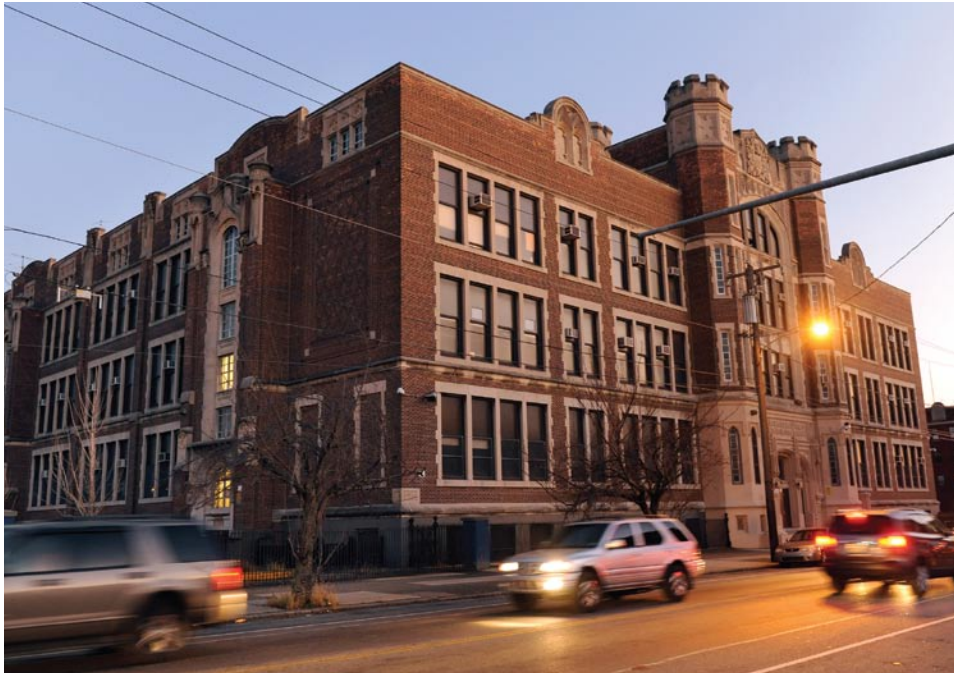
The former West Philadelphia High has been approved for sale for $6 million to a developer who plans to convert the buildings into 300 market-rate apartments. The site is located near the University of Pennsylvania.
