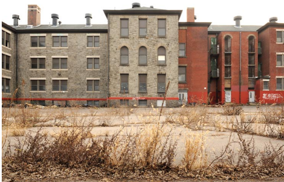
The Rudolph Walton School in the Strawberry Mansion section of North Philadelphia has been closed since 2003.
