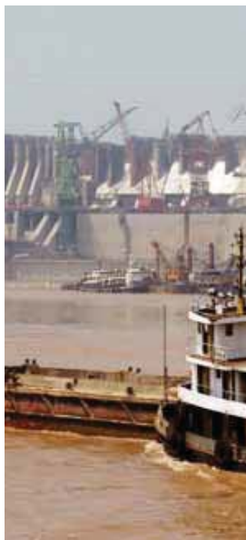
Construction of the Three Gorges dam on the Yangtze River
