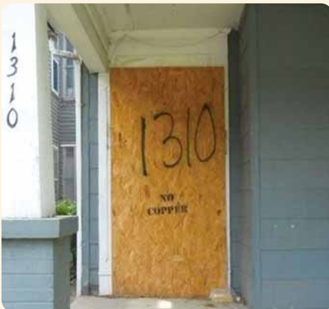
A vacant home in Louisville before the standard plywood board was painted.
