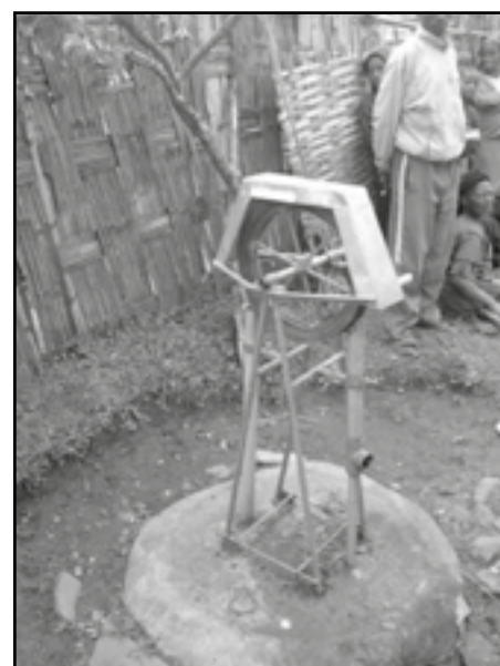
Figure 2.3 Chencha rope pump installed below ground level, and with no spout on riser pipe (Photo: Hailu, S.)
