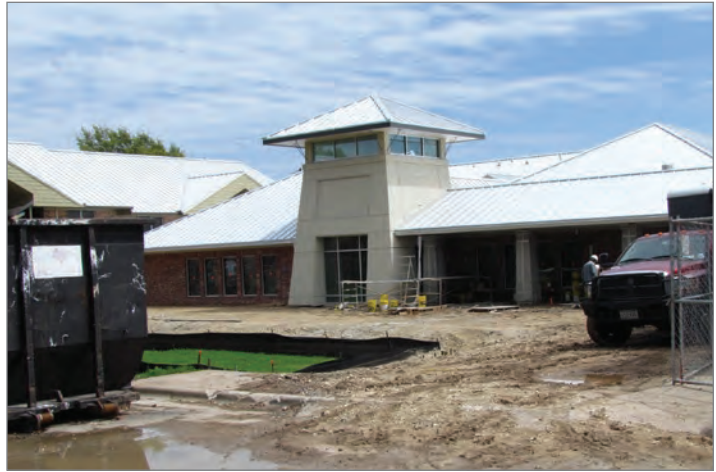
The Learning Center at Sierra Vista under construction.
