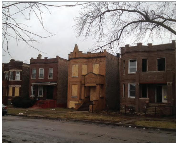
Row of dilapidated homes in West Humboldt Park.
