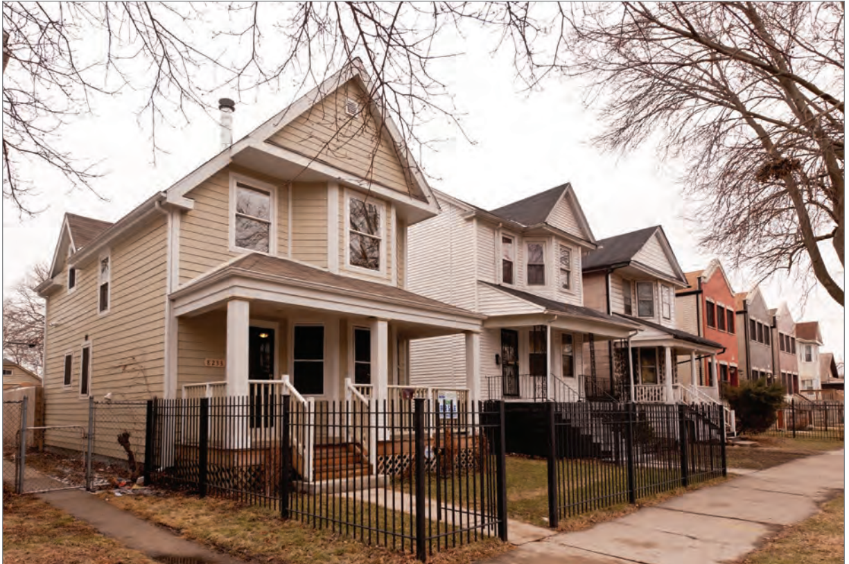
Exterior (above) and interior renovation (right) of a property.
