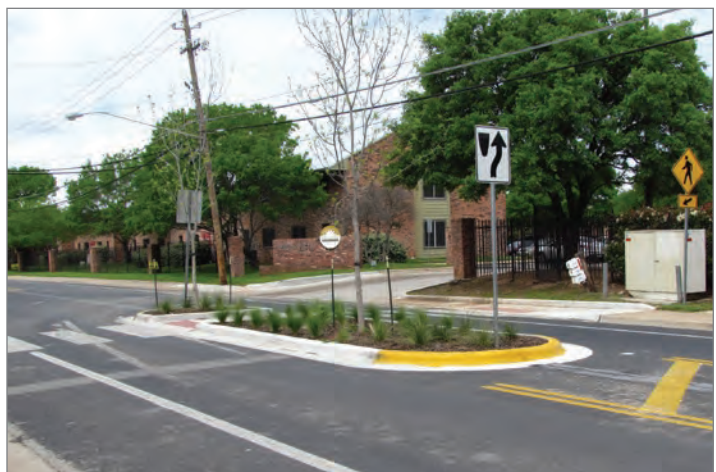
New traffic calming installation.
