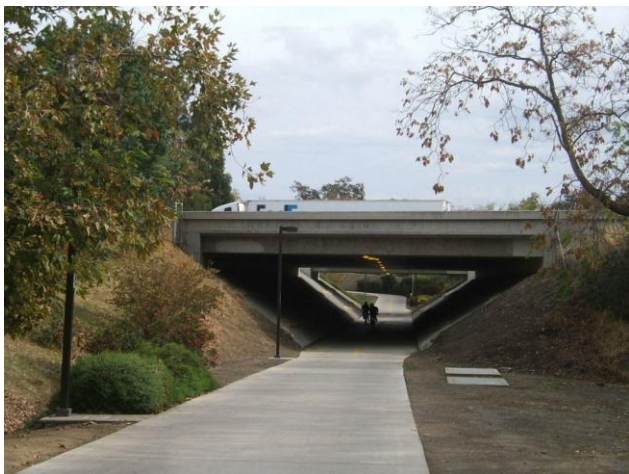
Figure B-7. Interstate 80 Undercrossing in Davis, CA
