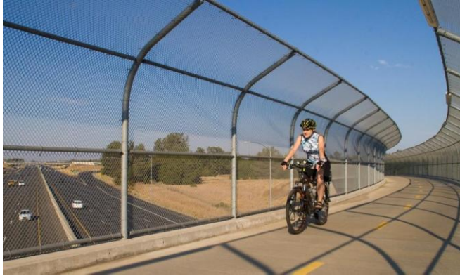
Figure B-6. Highway 50 overcrossing
