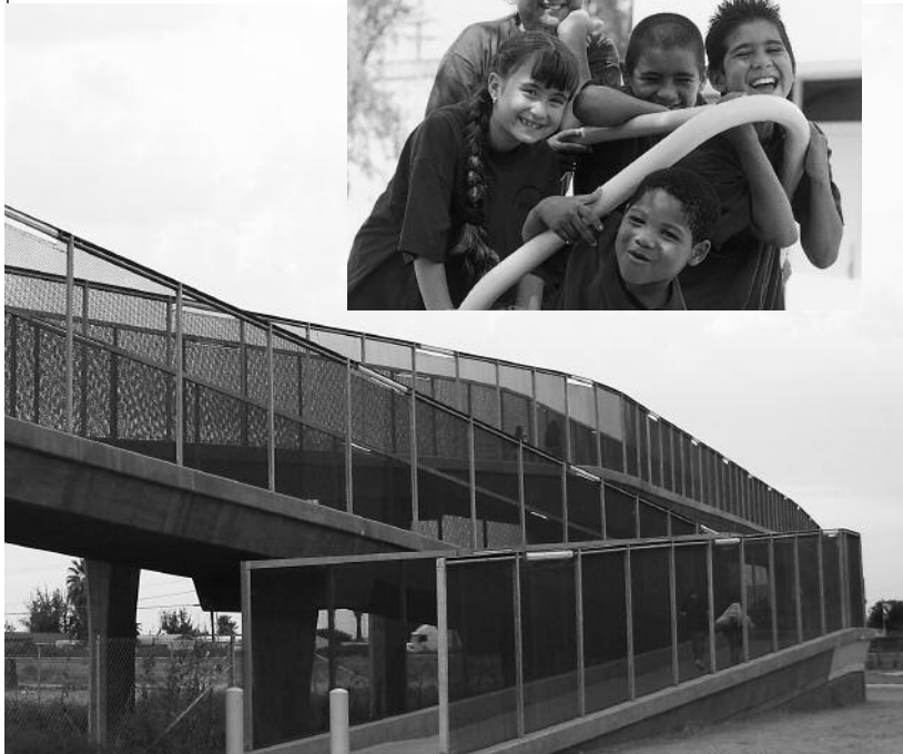
Since the sunset of TCWF's CYCHI, the community of Goshen has seen the construction of a pedestrian crossing that allows children to cross over the freeway to get to school. This need was identified during the life of the initiative by the community's Wellness Village, led by Community Services and Employment Training.
