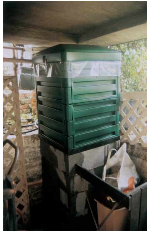
Downspout disconnections are a simple and inexpensive way for a homeowner to reduce polluted runoff. Here, a roof leader has been discretely routed under a porch to drain (left) into a concealed rain barrel (right) and mounted on cinder blocks to facilitate garden irrigation.
