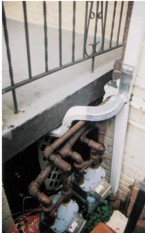
Downspout disconnections are a simple and inexpensive way for a homeowner to reduce polluted runoff. Here, a roof leader has been discretely routed under a porch to drain (left) into a concealed rain barrel (right) and mounted on cinder blocks to facilitate garden irrigation.
