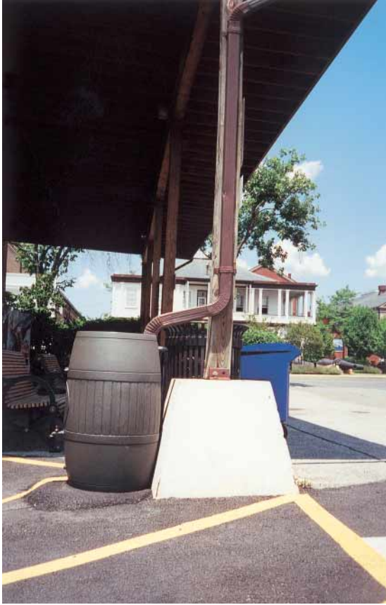
Rain barrels and cisterns are simple and inexpensive techniques to trap, store, and reuse stormwater for efficient landscape irrigation.
