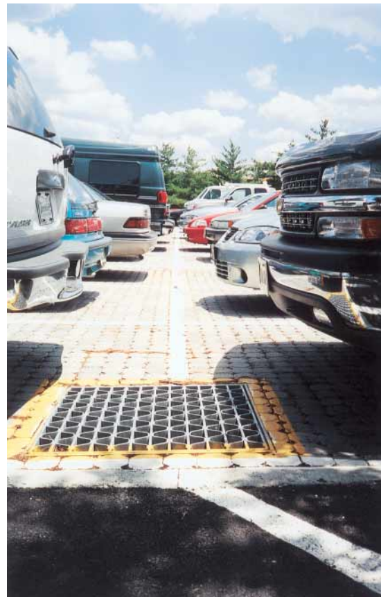
Strategic grading and use of pervious pavement as shown here in the Washington Navy Yard can be used effectively to treat and infiltrate parking lot runoff.
