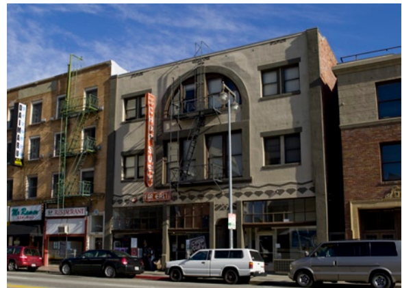
The Far East Building was rehabilitated by the Little Tokyo Service Center in 2003, preserving an important historic resource while providing sixteen new units of affordable housing. It is a contributing property within the Little Tokyo National Register Historic District. Experts in community and ethnic history can make valuable contributions to the citywide context statement by locating buildings and sites important to the history of a particular ethnic group or community. Photo: Emile Askey.
