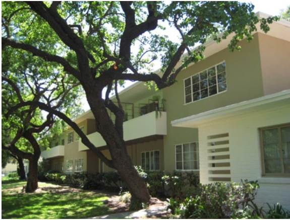
A view of Village Green (HCM #174). The Landmark Watch neighborhood group provided information on Clarence Stein's significant planning and design features for the Baldwin Hills Village garden apartment complex (now known as Village Green) that was instrumental in securing National Historic Landmark designation for this complex. City Council offices, city departments, Neighborhood Councils, and local organizations can provide valuable information to the citywide survey. Photo: Courtesy of Steven Keylon.
