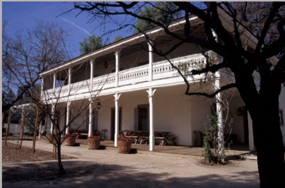
The Leonis Adobe in Calabasas (HCM #1), seat of an important 19th-century San Fernando Valley sheep ranch and one of Los Angeles's many significant historic sites. In 1962, it was the first building to be designated as an HCM by the newly formed Cultural Heritage Commission. Visiting historic places is a leading activity for cultural tourists. Photo: Gail Ostergren.
