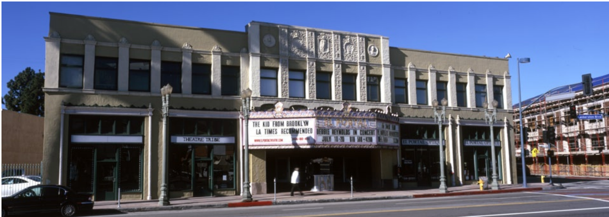
The El Portal Theatre in the North Hollywood Arts District (HCM #573). Identified as significant in a Los Angeles CRA survey, this historic theater was renovated and put back into productive use as a live-performance venue. The project served as a catalyst for economic development, including the renovation of additional historic structures along Lankershim Boulevard, North Hollywood's historic commercial strip. Photo: Emile Askey.
