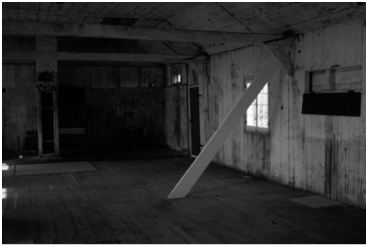
The interior of the east end of the Lazaretto, showing one of the diagonal braces as well as one of the windows modified for a late use of the building.
