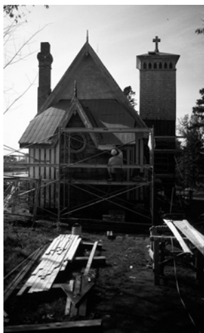
Figure 10. The Anglican Chapel. Built in 1877–78 (location 11, fig. 3), the Anglican Chapel was made of wood and set on masonry pillars. It was intended for the use of the staff and residents of the island, not for the immigrants. In order to preserve the structure's largely original appearance and to stop leaks, the pillars are being reinforced; a moisture barrier is being placed between the interior walls and the board-and-batten exterior skin; and the tin roof is being repaired.
