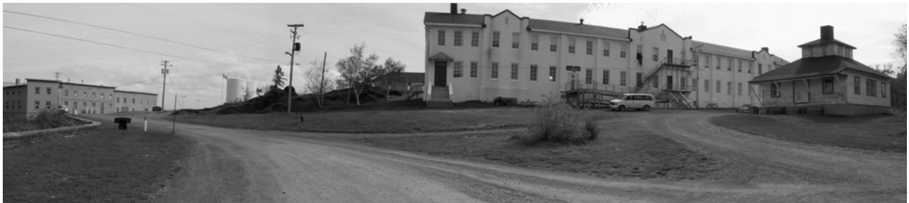
Figure 14. Third Class Hotel and the Bakery. The Third Class Hotel, built in 1914, is the largest of the three hotels, designed to hold 140 beds in its fifty-two rooms. Built of concrete, it included kitchens and dining areas at either end of each floor of the building, with living quarters in the center. While it offered close quarters and little privacy, it was fitted
