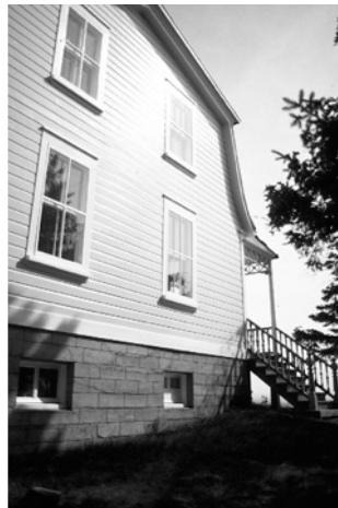
Figure 10. The Anglican Chapel. Built in 1877–78 (location 11, fig. 3), the Anglican Chapel was made of wood and set on masonry pillars. It was intended for the use of the staff and residents of the island, not for the immigrants. In order to preserve the structure's largely original appearance and to stop leaks, the pillars are being reinforced; a moisture barrier is being placed between the interior walls and the board-and-batten exterior skin; and the tin roof is being repaired.
