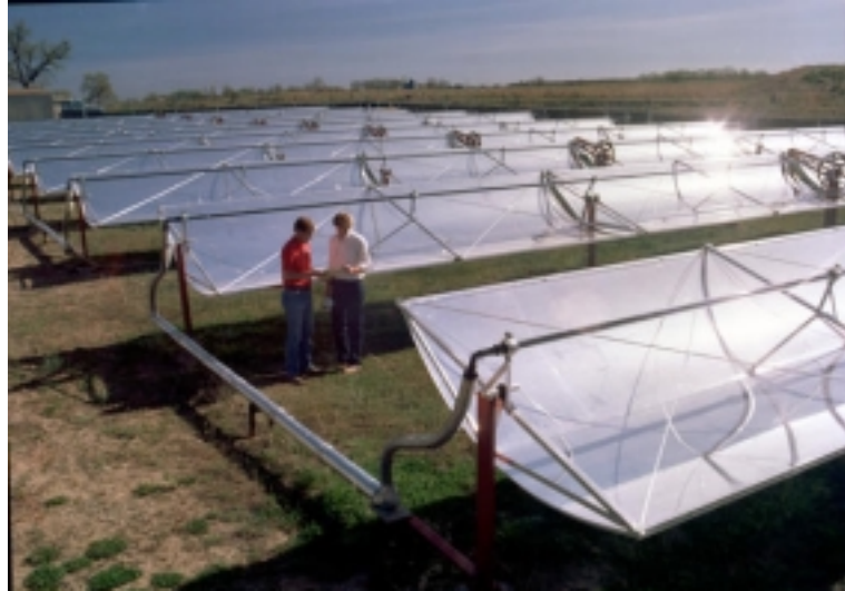
Parabolic troughs turn sunlight into power for Southern California.
