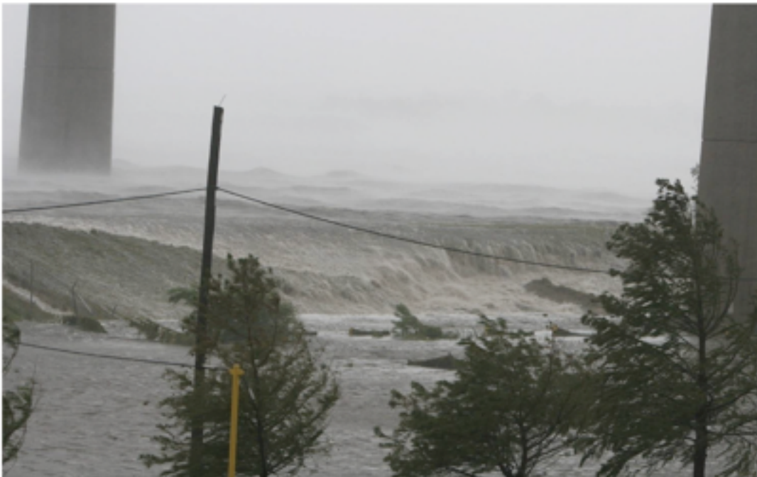
Figure 16. Storm Surge of Hurricane Katrina Amplified by Levees in the “Funnel”
